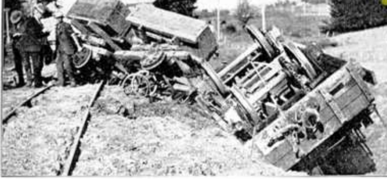
TWO MEN INJURED IN A RAILWAY ACCIDENT AT MAHIA, BETWEEN PAPATOTOE AND PAPAKURA. While working on the duplication of the line from Papakura to Papatotoe, this donkey engine and rake of trucks capsized over an embankment after leaving the rails near Mahia station. Two men received injury, one being seriously scalded.
